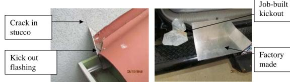
Above photo, left, shows existing flashing; above photo, right shows examples of job-built flashing such as found on this home compared with factory built flashing
