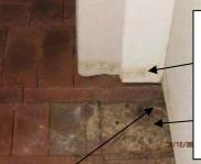
Brown staining and brown glue from deteriorated osb substrate
