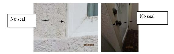
Next best seal is a well-kept properly applied caulk seal using good caulk, such as NP1. The existing caulk on the dissimilar materials of this home was in poor condition where found and some areas were not caulked.
