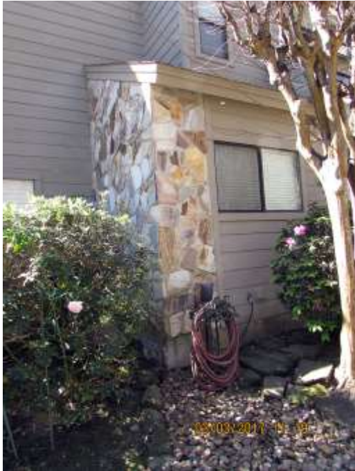
Laundry room exterior
